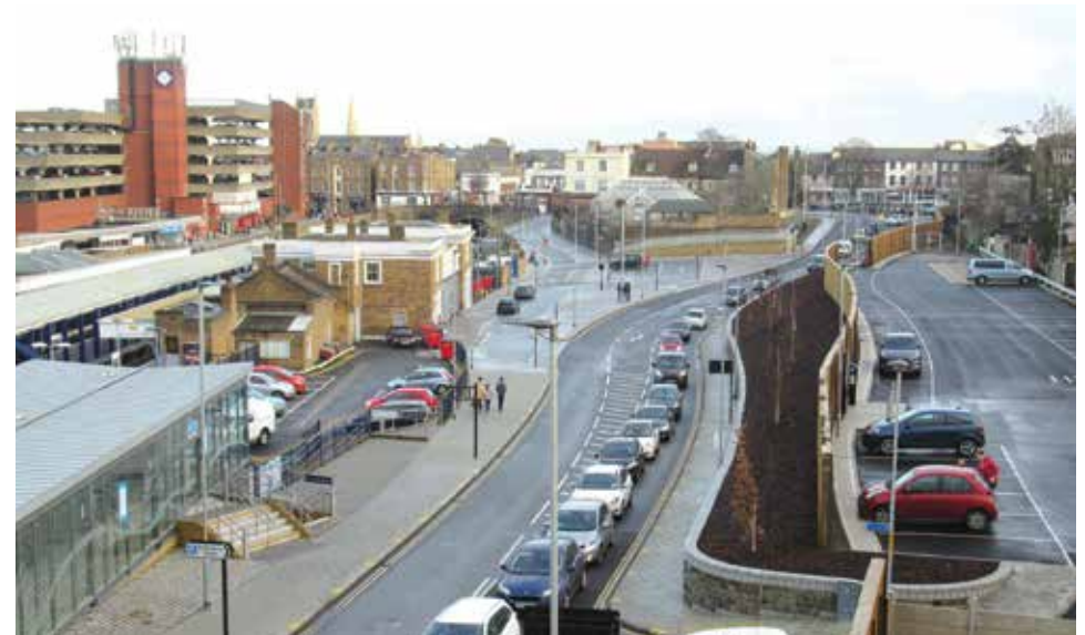
Rathmore Road completed improvements in Gravesend
